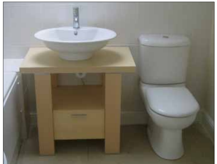
▲ Bathroom renovation – bespoke shower/sink and toilet plumbing/tiling
